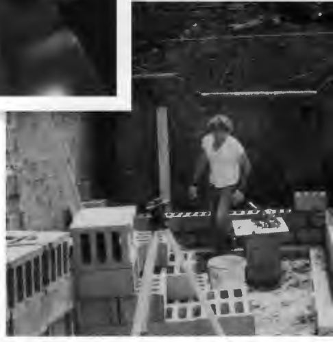
Don laying cement blocks for Music Room (Photo by Ben Robertson)
